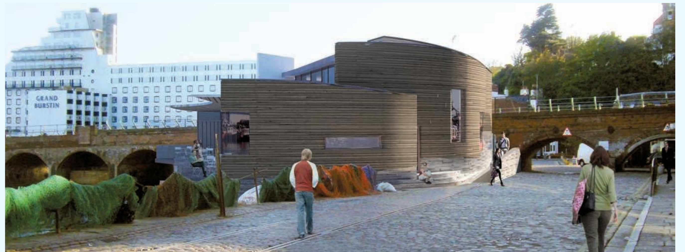
The street facade, which features three curved walls, is clad in horizontal charred timber.
