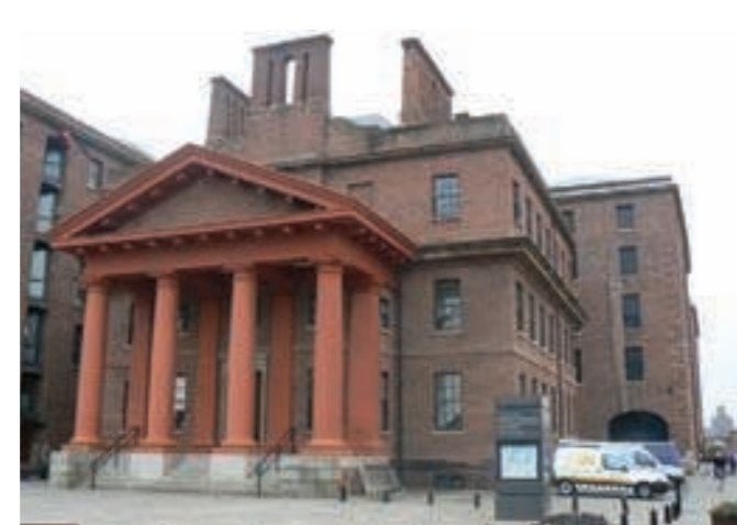
The grade I Dock Traffic Office.
